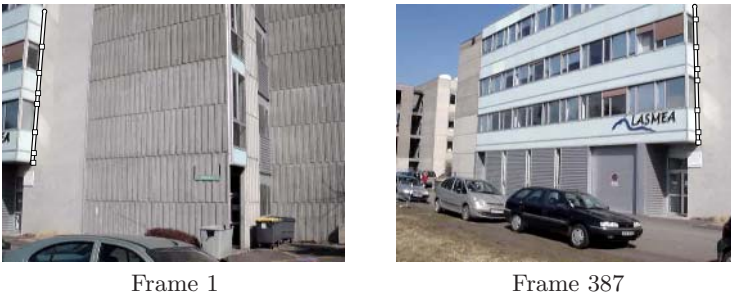
Fig. 5. 2 out of the 387 images of the ‘building’ sequence, overlaid with the matching segments and 7 corresponding points
